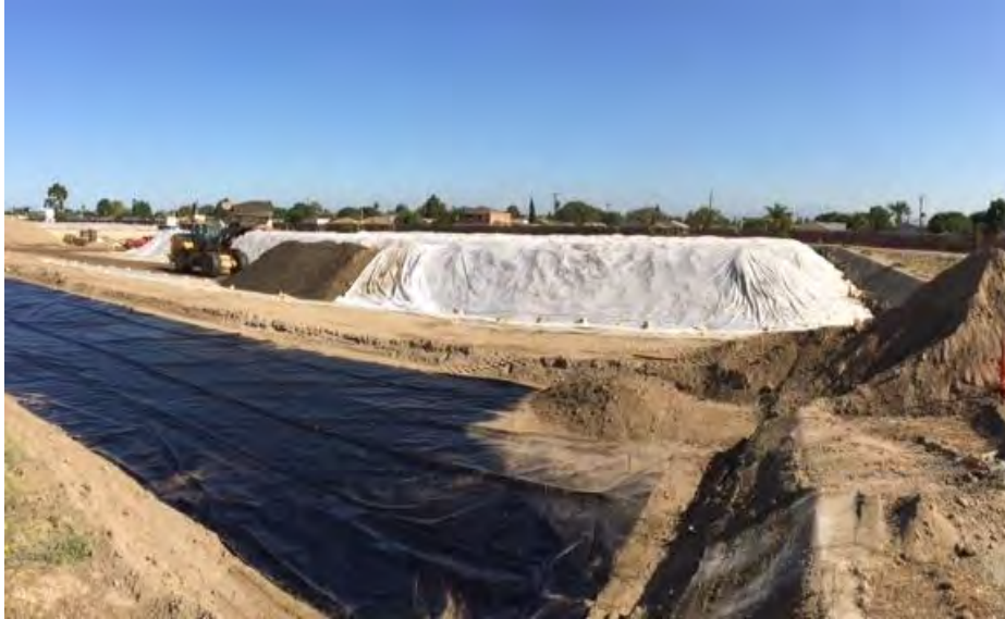
Photo 7: Liner emplacement under treatment stockpile.
