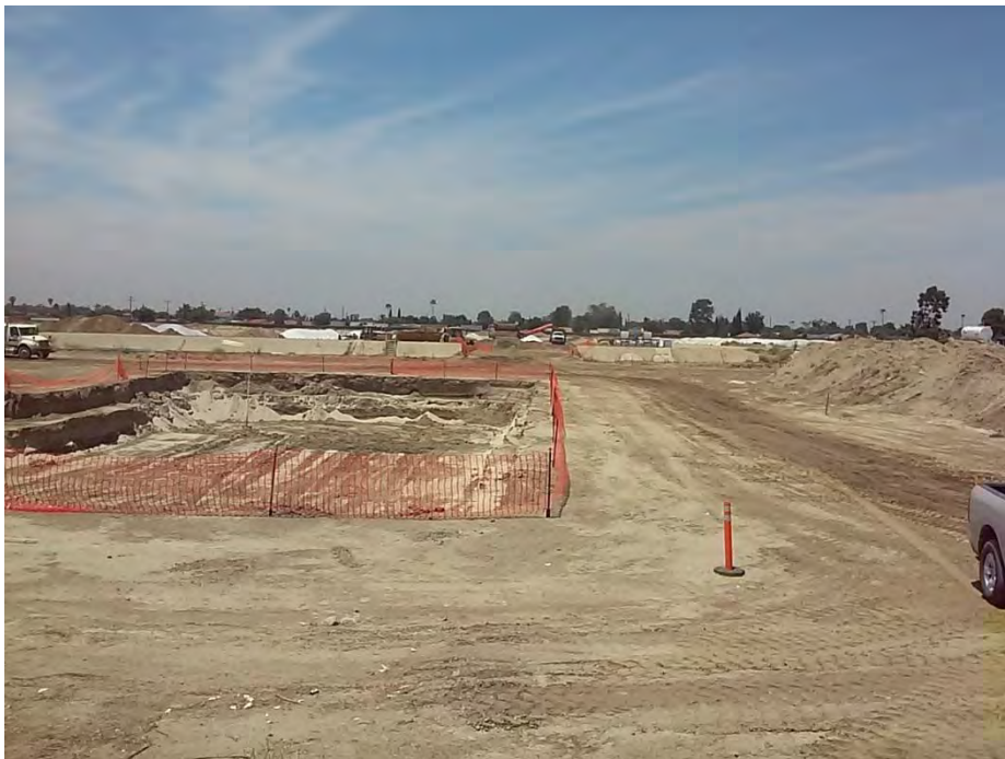
Photo 6: Example photo of Excavation (Excavation #2).
