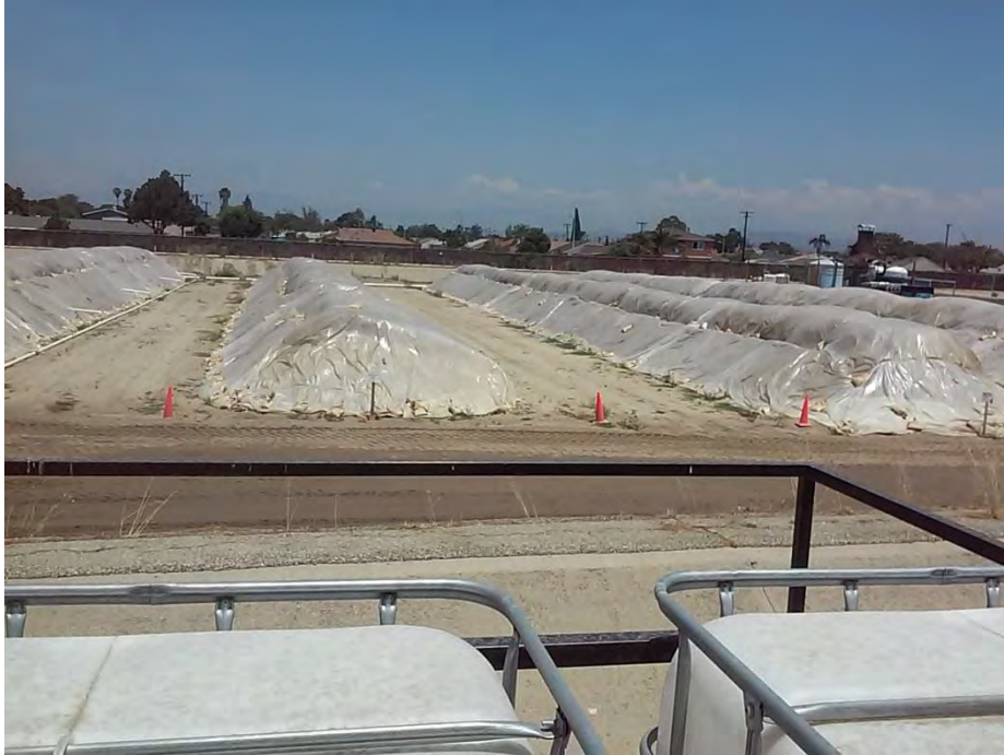
Photo 5: Soil Treatment Piles.
