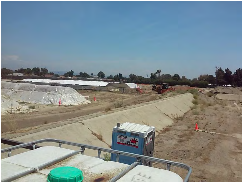
Photo 4: Soil Treatment Piles.
